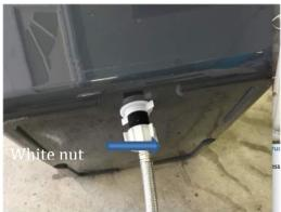
Note the connection between level control valve and connector, which is in turn connected to the customer's garden hose. The white nut indicated by the blue arrow must be tight. No leaking from the Reservoir permitted or nutrients are lost.
